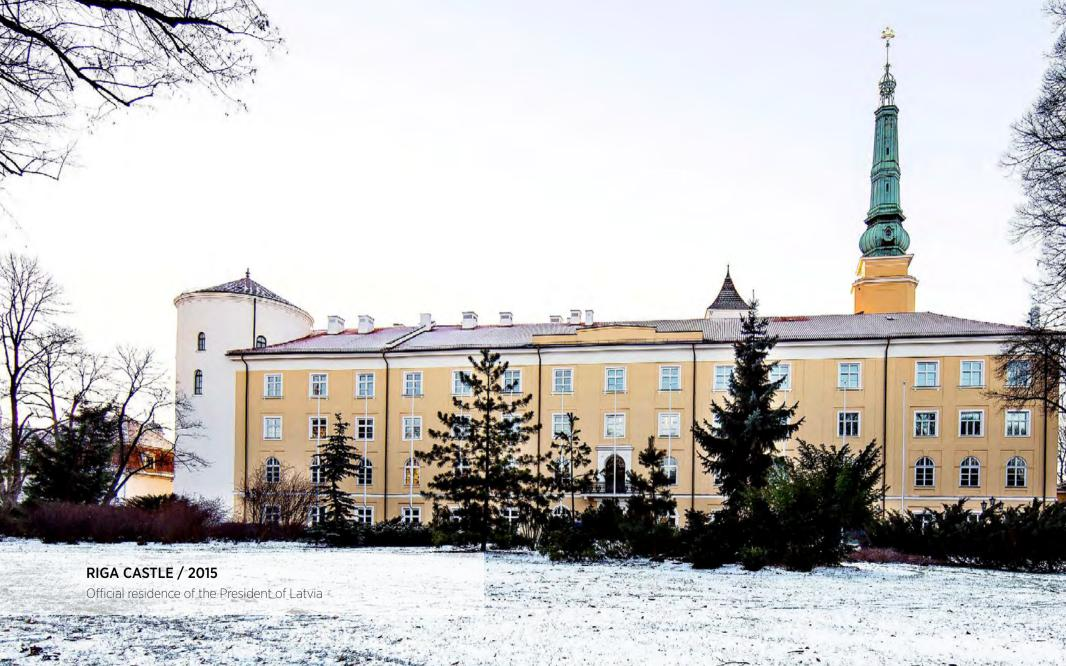
Reconstruction of Riga Castle premises comprised both functional and artistic reconstruction in all out of 8959.2 m<sup>2</sup>. Reconstruction itself involved reinforcement of the basic support structures and foundations, including renovation of the interior finish.
